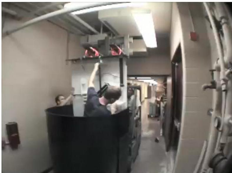
Photo of main switch assembly being lowered into switch tank
